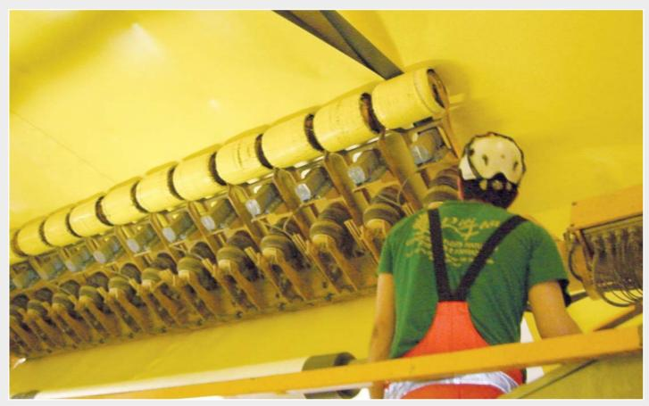
Mechanical application of the prefabricated, 4.30 m wide plastic sealing sheets onto the Velcro-backed discs located below. Welding is then carried out.
