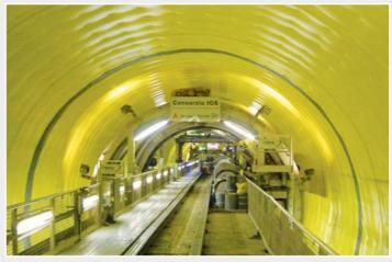
Finished tunnel seal. The individual sheets are welded in parallel.
