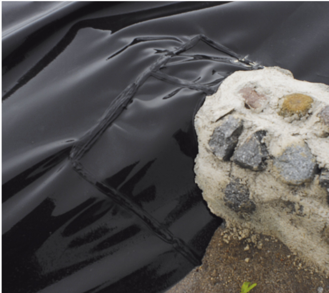
The HDPE membrane as it is seal welded to the slurry line. Welded with the WELDPLAST 3C hand extruder.
