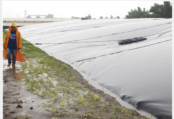
Cesspool filled with methan.
