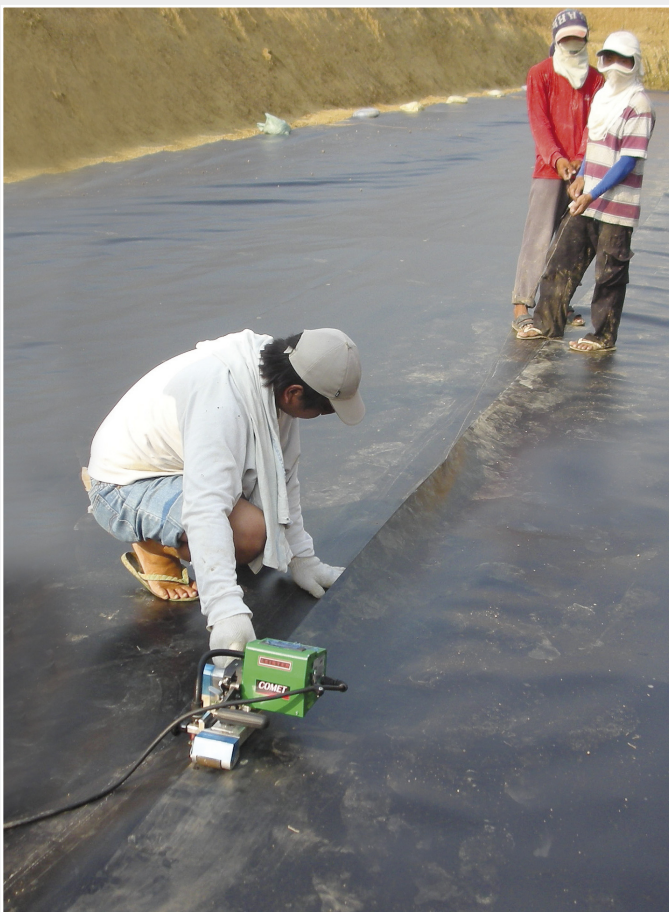
The COMET unit welding the HDPE sheets.
