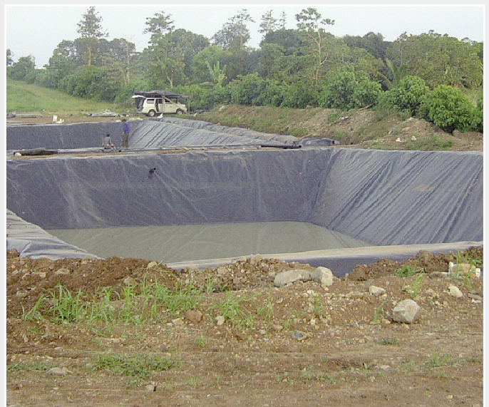
The basins, some 4000 m 2 in size, before being filled with slurry.
