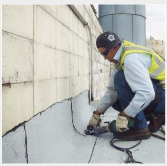
The powerful ELECTRON with wide slot nozzle for welding intricate details.
