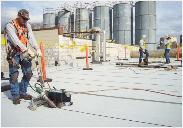
Safe and secure welding of bitumen sheeting with the BITUMAT B2.
