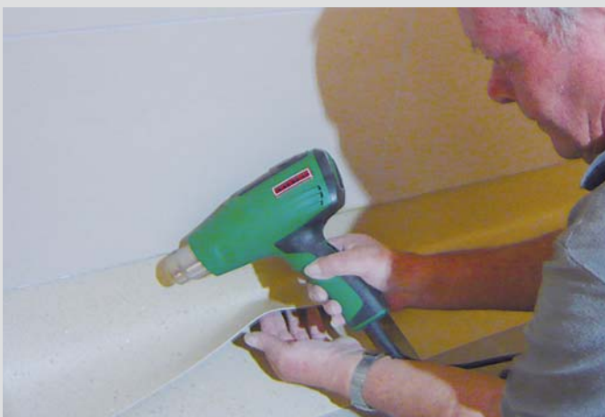
Rapid shaping of floor coverings
